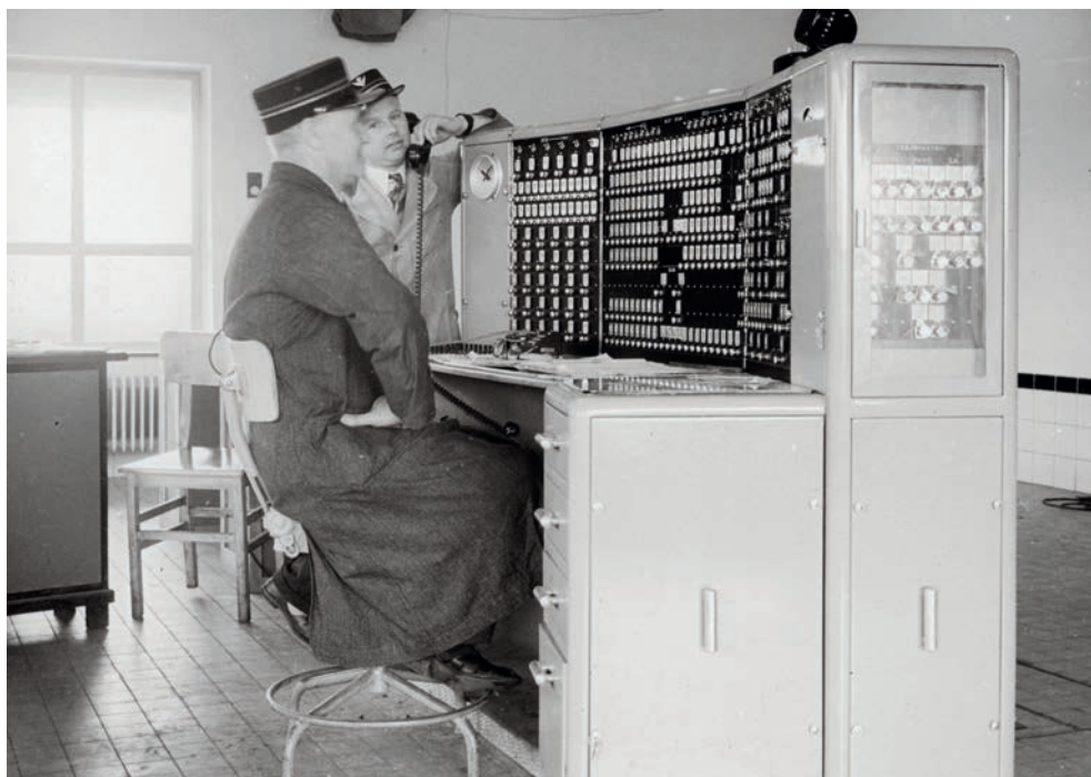
FIG. 2 Al-relaisgestel in blokpost 15 te Aalst, 1954 (Brussel, Archiefdienst en Fototheek NMBS-Holding, Z03831c, seinhuis Aalst-interieur (1954)). Al-relay system in signal box 15 in Aalst, 1954.
