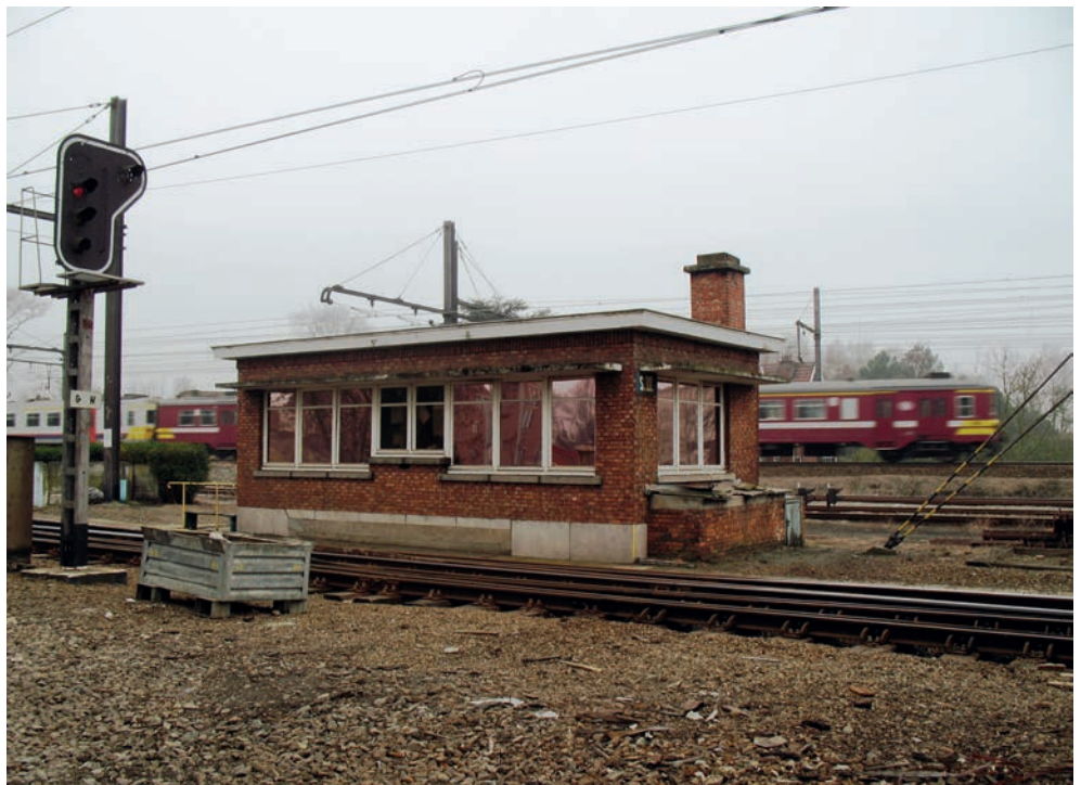
FIG. 5 Seinhaus IV in Aalst, 1956-1957 (foto Laura May, 17/03/2011). Signal box IV in Aalst, 1956-1957.
