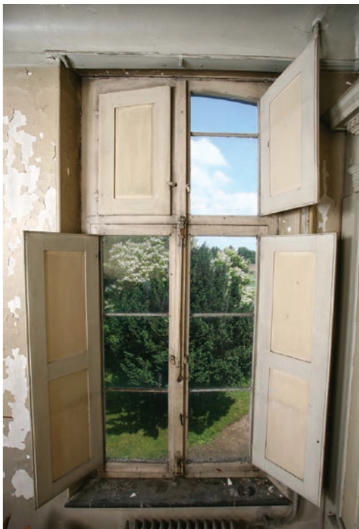
FIG. 38 Venster in vertrek 131 (oostvleugel). Window in room 131 (east wing).
