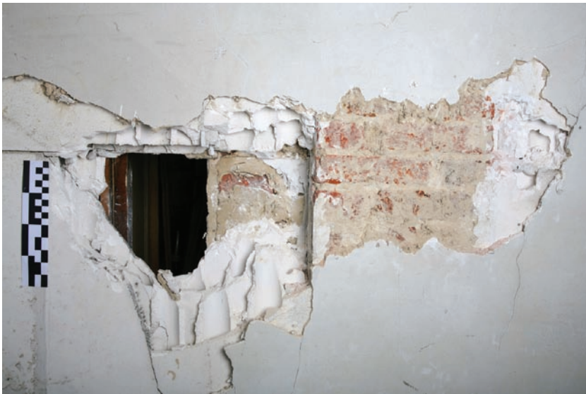
FIG. 22 Bakstenen dwarsmuur tussen de vertrekken 128 en 129 (oostvleugel), gezien vanuit de middengang. Transverse wall in brick between the rooms 128 and 129 (east wing), seen from the central hallway.
