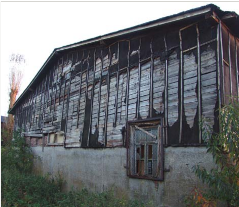
FIG. 12 Foto van de westgevel van de kleine barak, toestand december 2007. Photo of the western elevation of the smaller barrack hut, in its December 2007 state.
