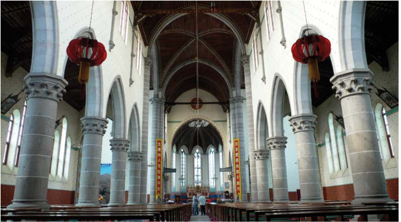
FIG. 25 Church of Xuanhua, interior view to the north (© THOC, May 2011).
