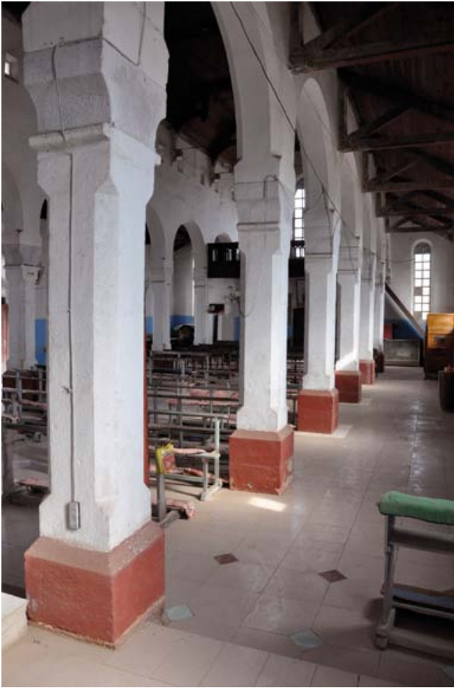
FIG. 19 Church of Shebiya, piers of the nave and western aisle (© THOC, May 2011).
