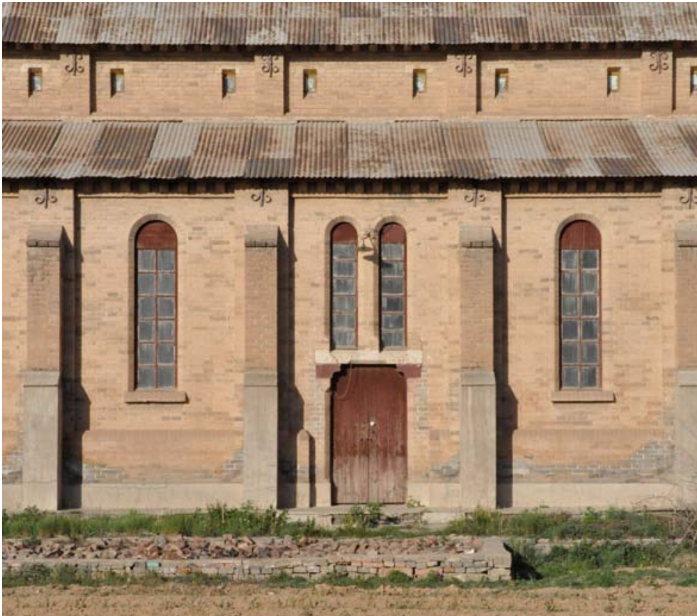
FIG. 18 Church of Shebiya, detail of the brickwork of the western façade (© THOC, May 2011).
