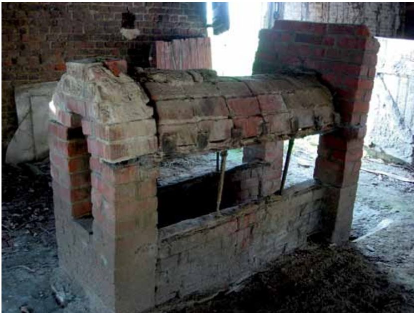
FIG. 14 Eestoven in de hopast Russen in Poperinge. Drying kiln, oast house Russen in Poperinge.
