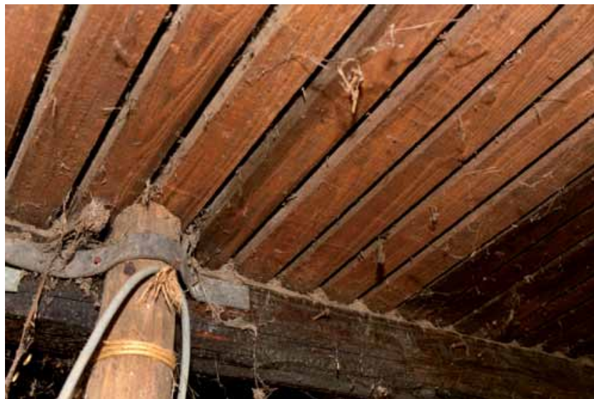
FIG. 27 Eestvloer met platte houten latten in de hopast Deheegher in Poperinge. Drying floor with flat wooden slats in hop oast house Deheegher in Poperinge.
