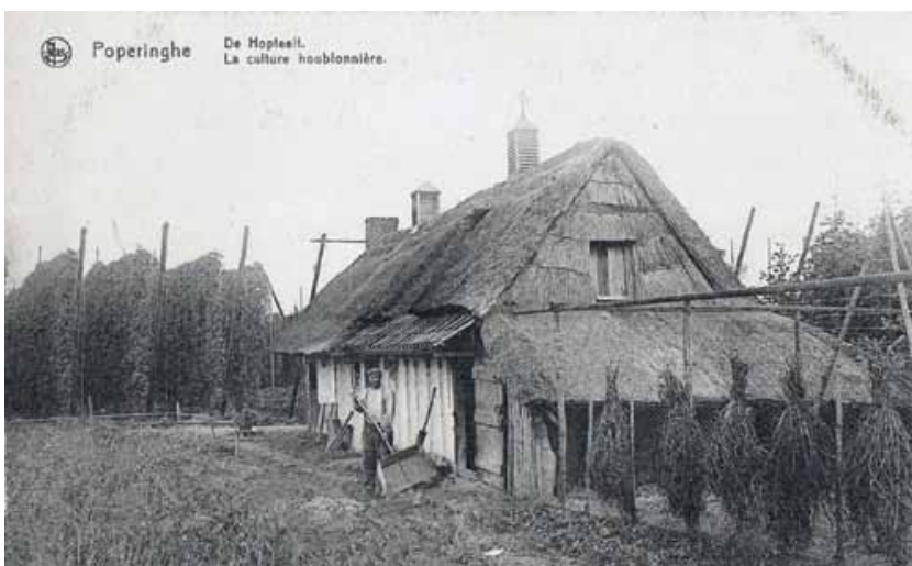
FIG. 24 Hopasten met houten dakruiters. Hop oast houses with wooden turrets.
