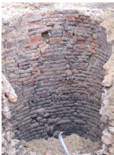
Afb 54 Detail baksteenverband waterput S496
