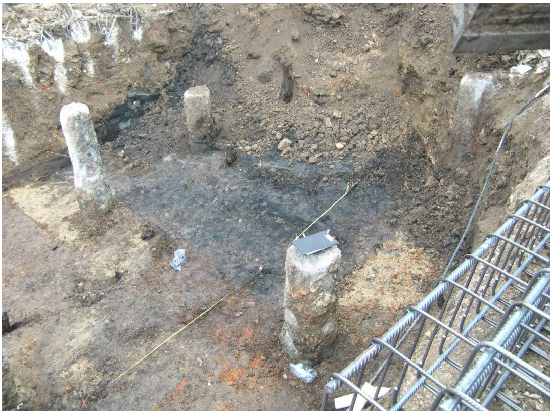
Funderingen in steenbakkerijafval
